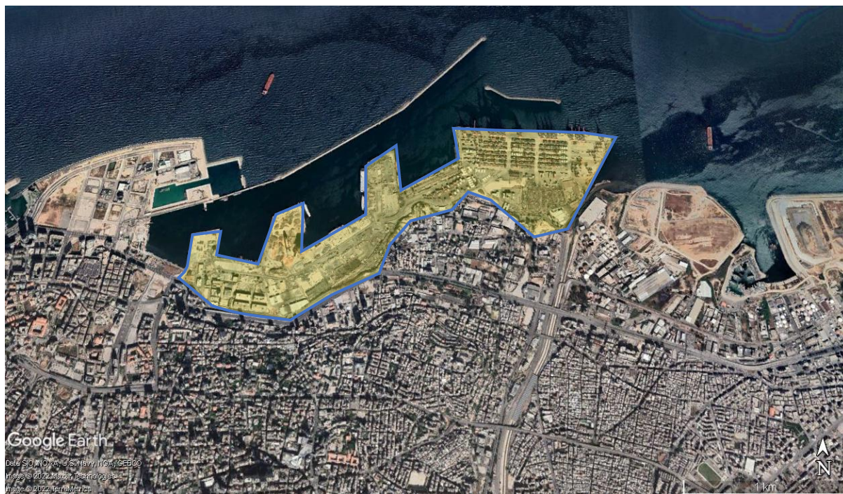
Figure 1: General Location of PoB (Google Earth Satellite Image, June 2022)
