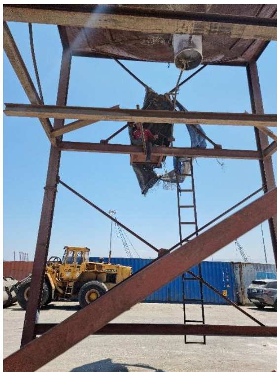
Figure 11: Operators sitting at heights are unprotected from falls and do not wear any kind of PPE 25.
