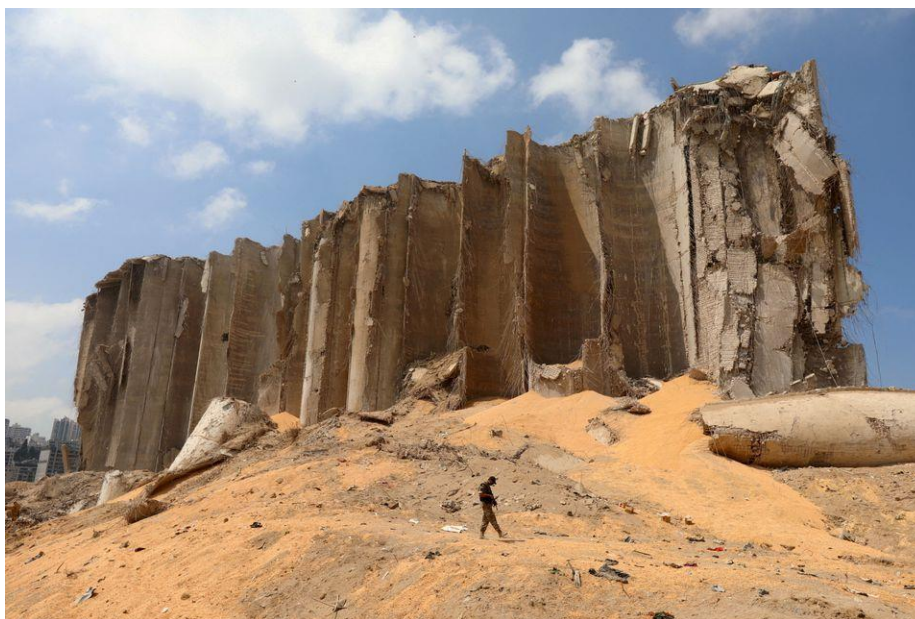
Figure 3: Damaged Silos at PoB after August 4, 2020 15
